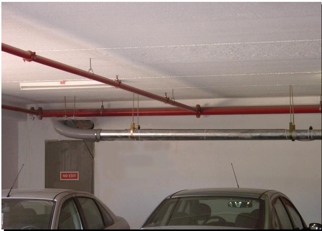
**An Electronic Security Pipe designed to protect video, data, telephone and communication cables against tapping.**
